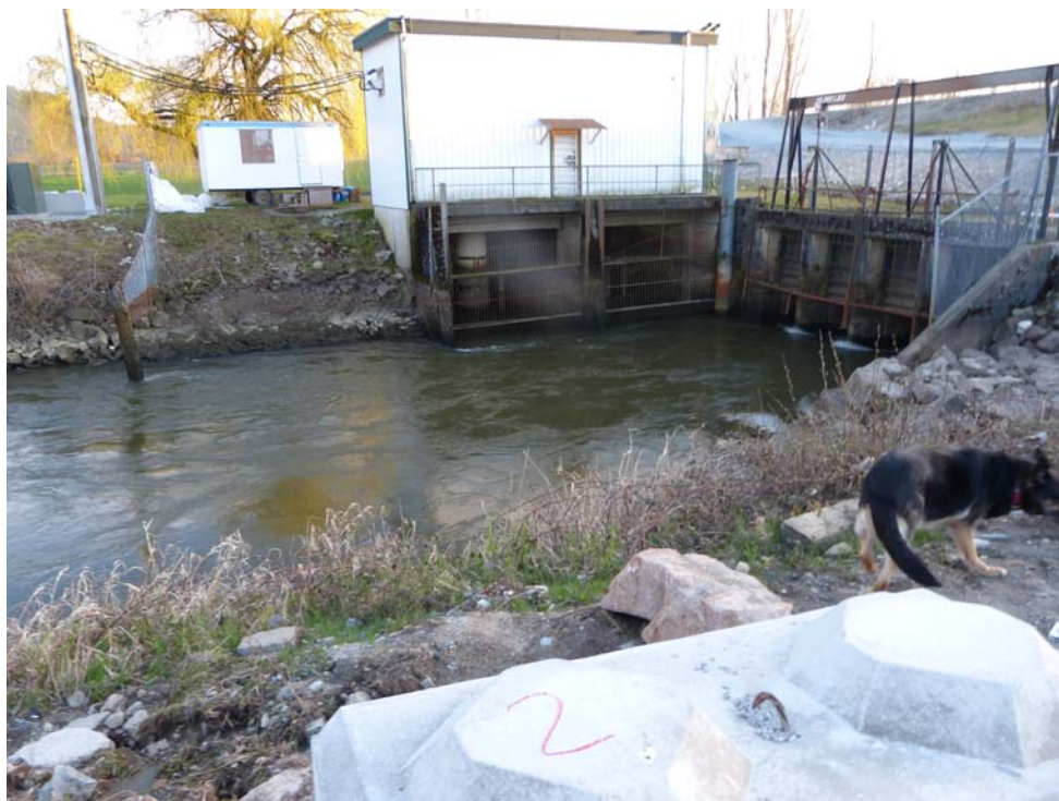
1949 pump house with flood boxes on the right side
