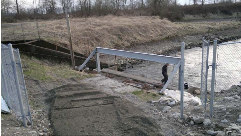
New flood gate control beam
